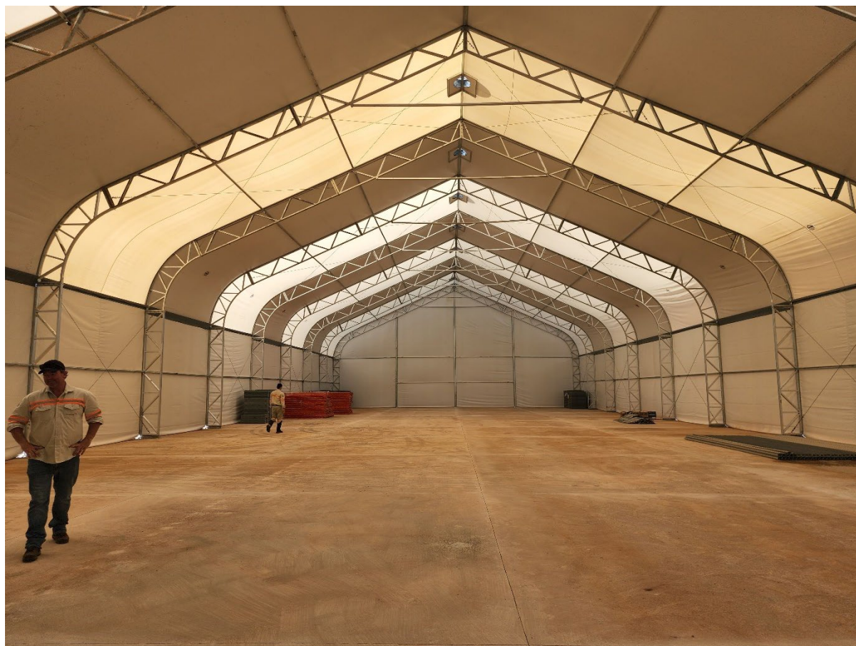
Figure 4: New Core Shed
