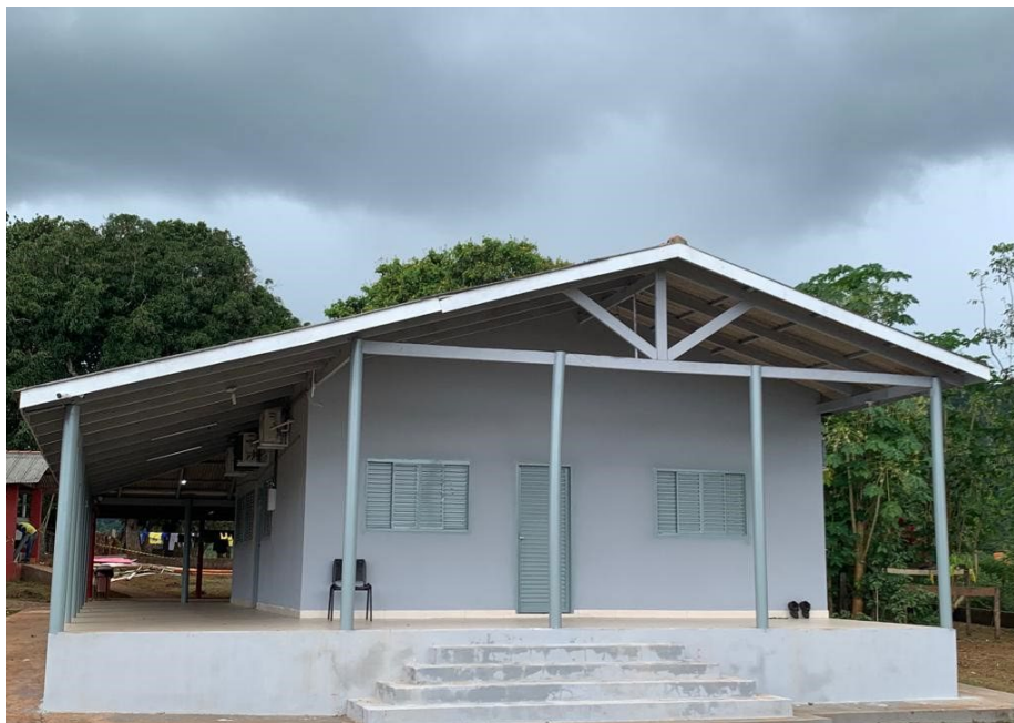
Figure 6: New On-site Accommodation at Jaguar
