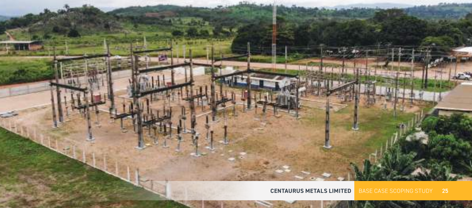
Figure 18 - 138kV National Grid connection at Tucumã
