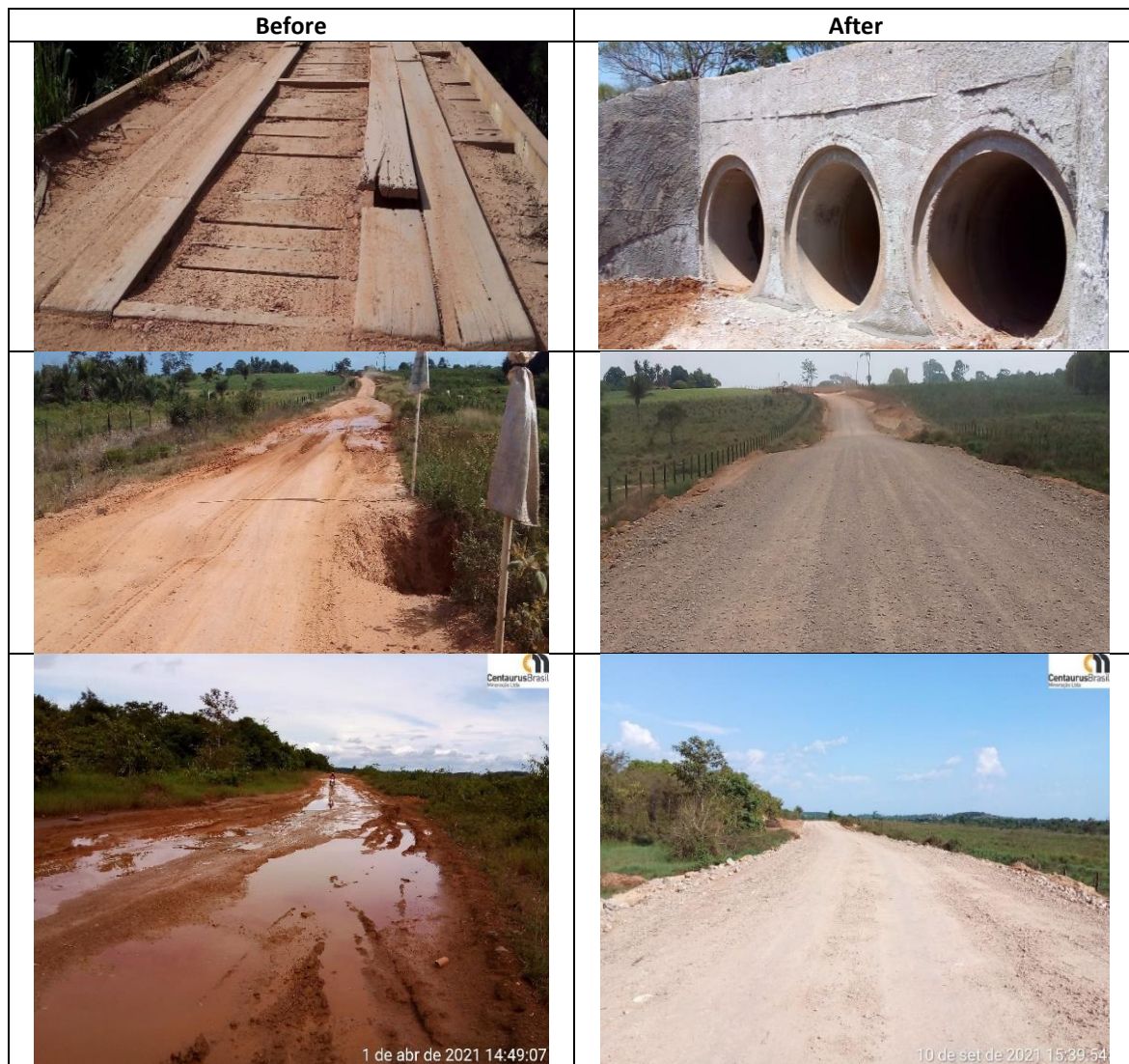
Figure 15 – Road Upgrade Work – Before and After
